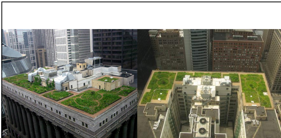
Chicago City Hall – the coolest place to be, thanks to this $2.5 million rooftop garden ( not open to the public – the 11-storey drop might have something to do with this).
