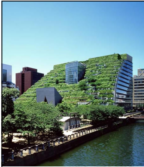
ACROS Fukuoka, offices under green terraces – Japan
